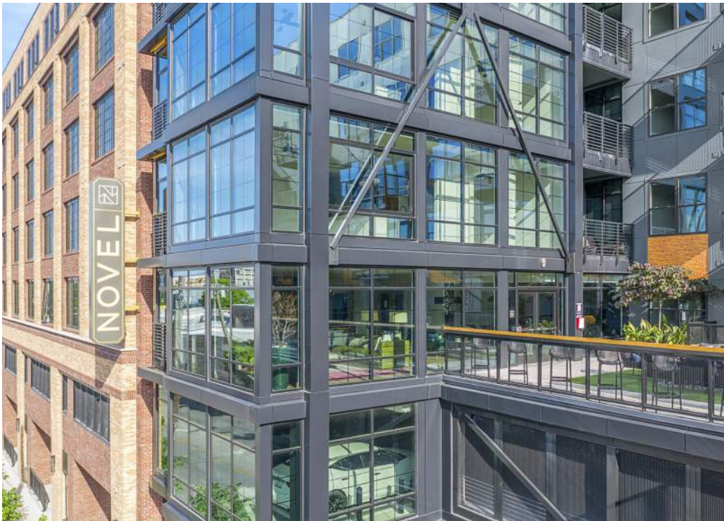
CROSS-BRACING: METAL PANEL + FIBER-CEMENT
